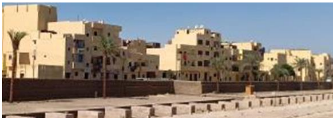
Fig. 26. Reducing the irregularity of skylines by raising parapets and building walls to complete upper floors (Photo credit: Authors)
