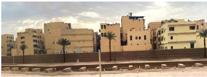
Fig. 25. Repainting and finishing of buildings using unified colours. (Authors)
