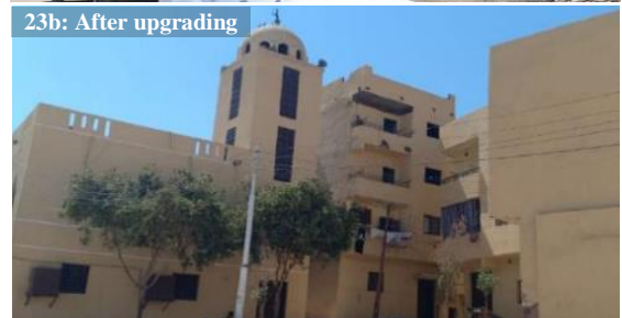
Fig. 23a and 23b. Building new parapets and walls to complete the missing parts (Photo credit: Authors)
