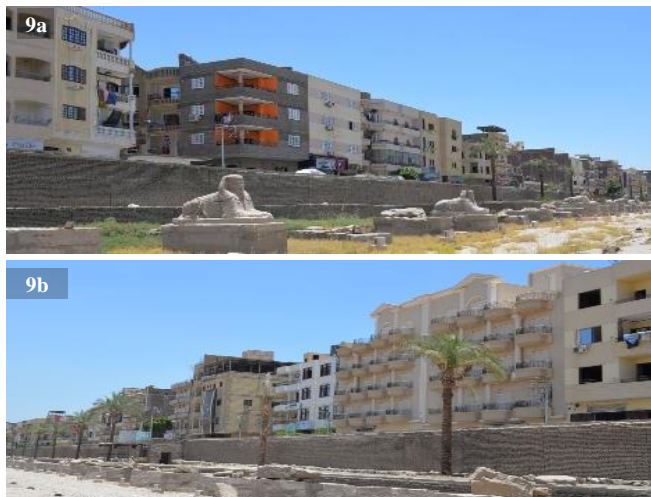
Figs. 9a and b: The buildings at the two sides of section "B" (Authors)
