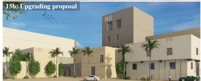
Fig. 15a and 15b. Adjusting skyline by raising heights of parapets and constructing walls between columns of incomplete upper floors. (Authors)
