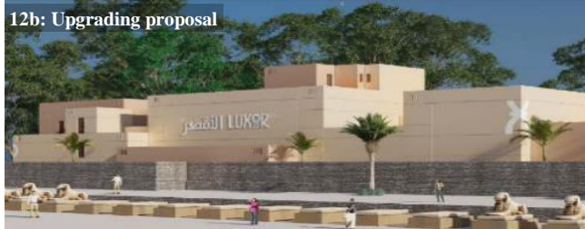
Fig. 12a and 12b. Removing crumbling walls and completing missing parts then plastering and painting of façades using unified colors (Source: Authors)
