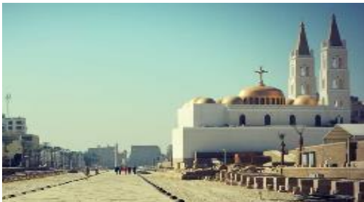
Fig. 30. St. Mary Church after renovation
