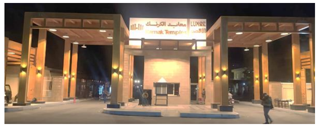
Fig. 21. The new gate to Karnak parking lot after execution
