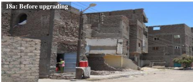
Fig. 18a and 18b. Removing crumbling walls as well as plastering and painting of unfinished façades (Sources: Authors)
